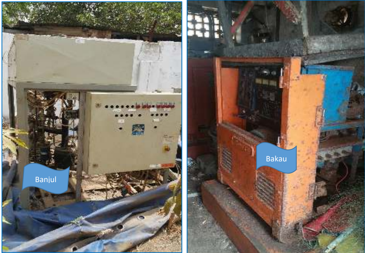
Picture 10: showing broken down or dilapidated ice plant machines in the CFCs
